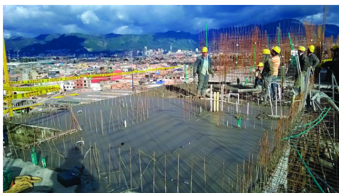
Instrumentation of a concrete slab for industrialized systems in order to determine maturity. The photo shows the thermocouples and the digital temperature recorder.
