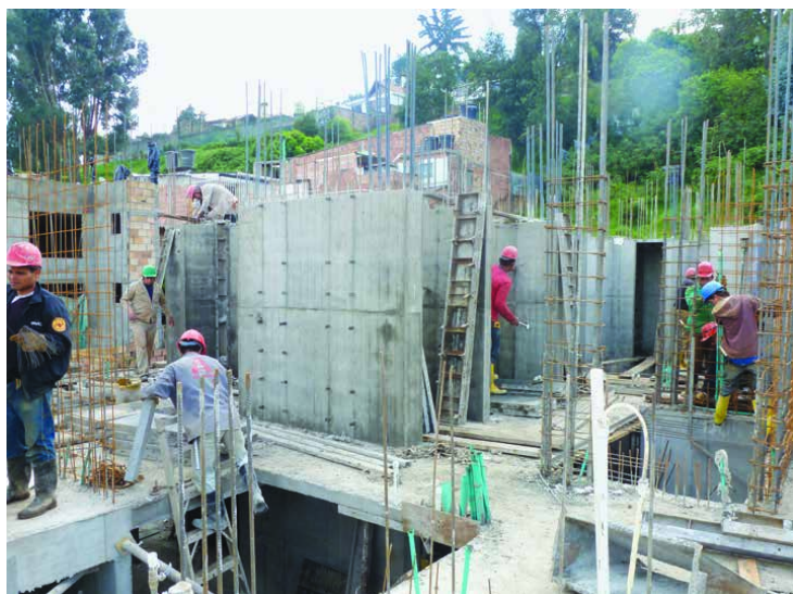
Building under construction using industrialized systems.
