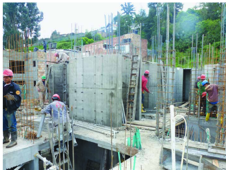
Walls and slabs built using industrialized systems.
